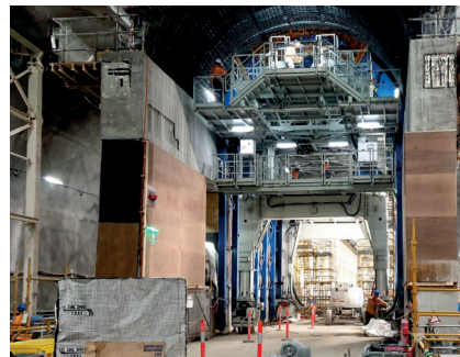
Tunnel formwork on site
