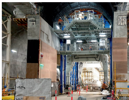
Tunnel formwork on site
