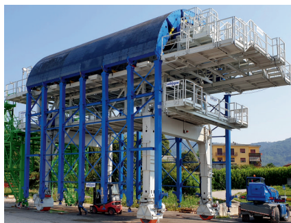
Adit shutter fitted on the tunnel formwork
