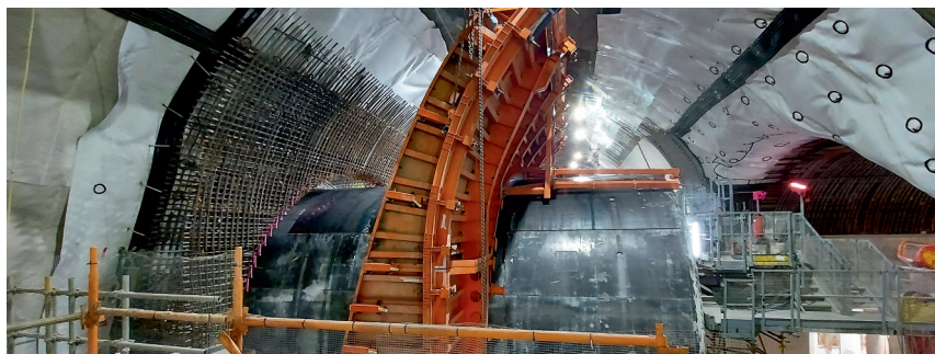
Adit shutter fitted on the tunnel formwork
