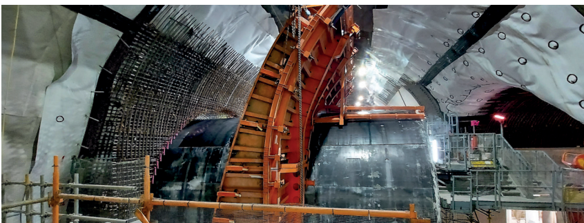
Adit shutter fitted on the tunnel formwork
