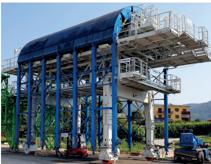
Adit shutter fitted on the tunnel formwork
