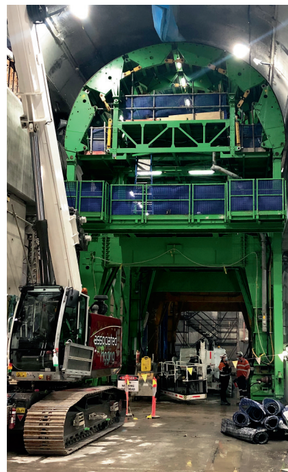
Tunnel formwork on site
