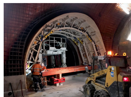
Collar formwork support
